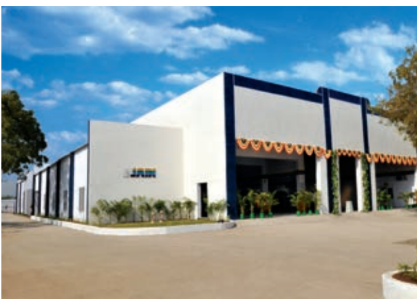
Drip and Sprinkler Irrigation Systems and Plastic Piping : Jain Plastic Park, Bhavnagar, Gujarat (India)
