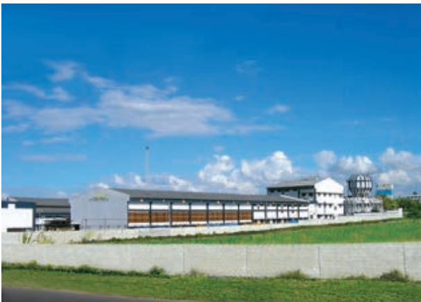
Drip and Sprinkler Irrigation Systems and Plastic Piping : Jain Plastic Park, Kondamadugu, Andhra Pradesh (India)
