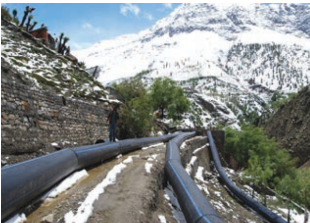
HDPE Pipe installed on the slopes of Himalayas
