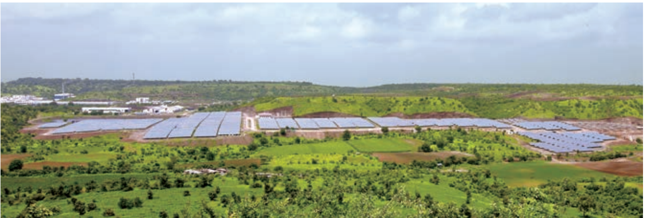
8.5 MW Solar power plant at Energy Park, Jalgaon.
