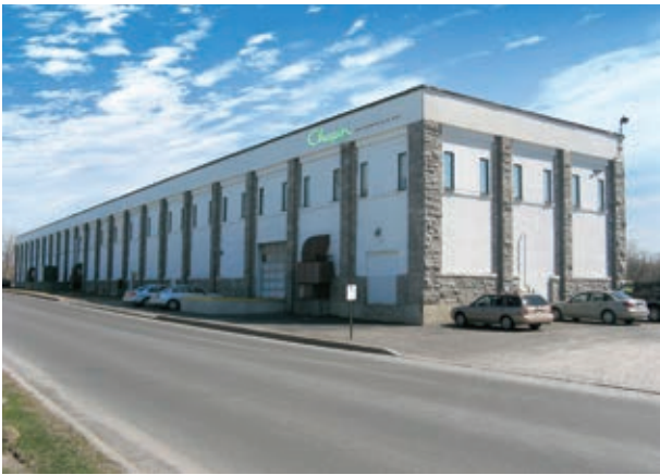
Drip Irrigation Systems : Jain Irrigation Inc., Watertown (USA)
