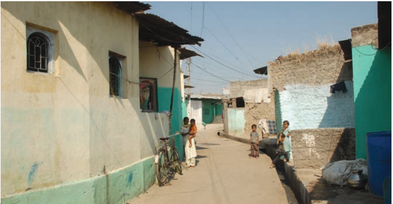
Concrete streets and drainage systems in Wakod, India
